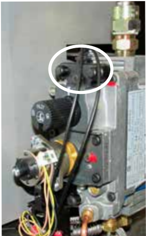
DC Sparker Wires
